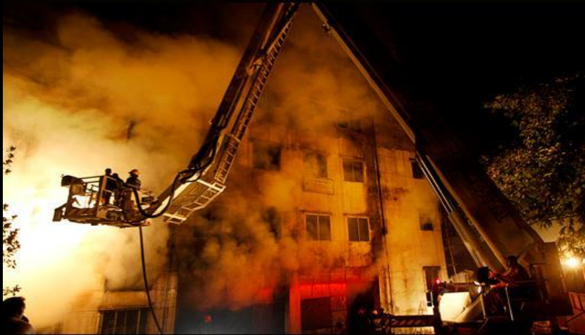
November 24, 2012 Tazreen Factory Fire Dhaka, Bangladesh
